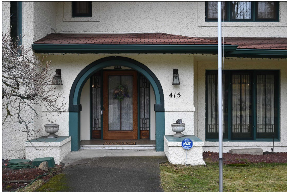
Front entry door showing mosaic, sidelights, and oak storm door
