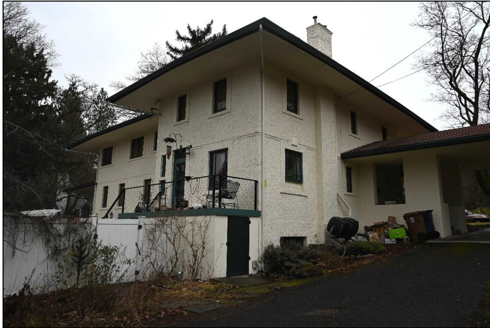
Rear (north) elevation, looking southeast
