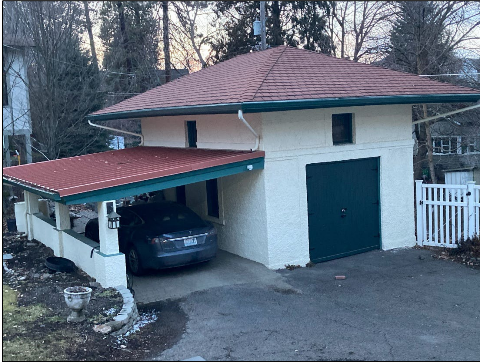
Garage and carport, looking northwest
